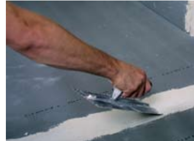
Tape all joints with fiberglass mesh tape or wedi waterproof tape or wedi polyurethane sealant and begin tiling!
