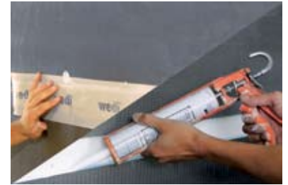
wedi polyurethane sealant or waterproof tape is applied on the seams and fastener points.
