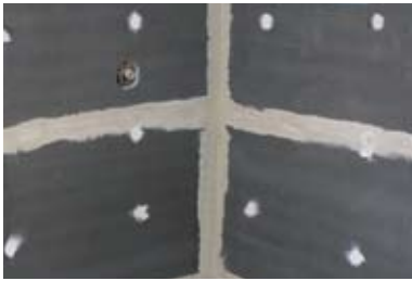
The shower is complete and ready to be tiled.
