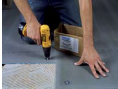
Fasten with wedi fasteners.
