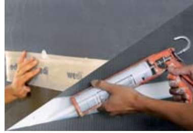
wedi polyurethane sealant or wedi waterproof tape is applied on the seams and fastener points.
